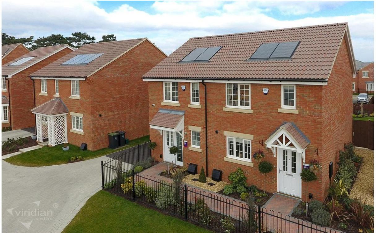
(Source: http://www.viridiansolar.co.uk/gallery-of-solar-installations.html#(grid|popup)=gallery/3096-TaylorWimpey-Raunds-Avonside(C)ViridianSolar.jpg ; accessed 29 th April 2019)
